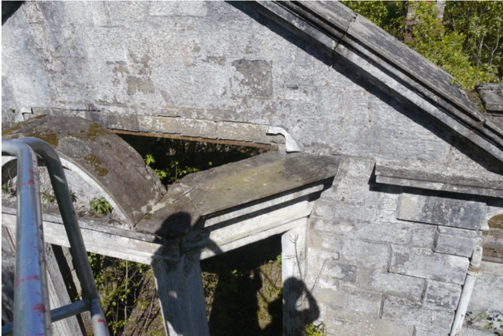
Above - rusted iron beam supporting pediment.
