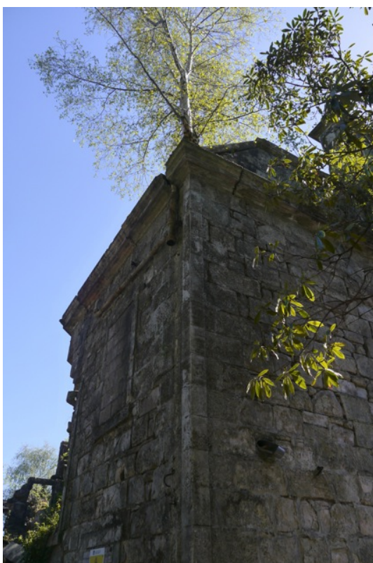
Above - vegetation growing off concrete second floor behind west gable. Left - open mortar joints to west gable.
