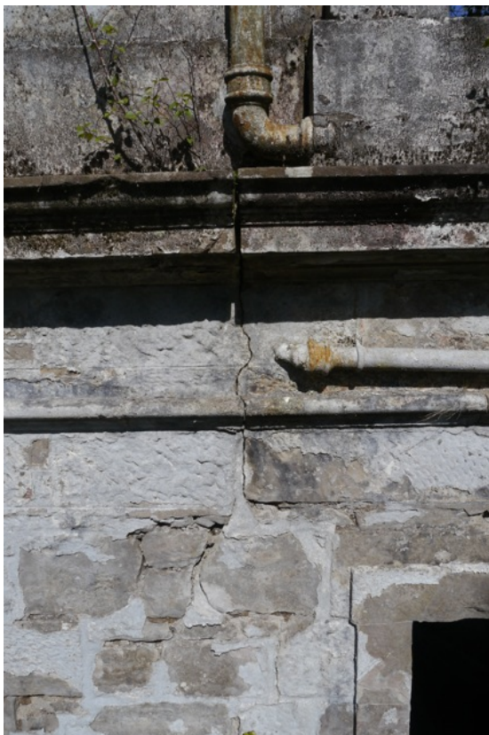
Below - Cracks and open joints to be repointed and plain wall areas lime rendered.
