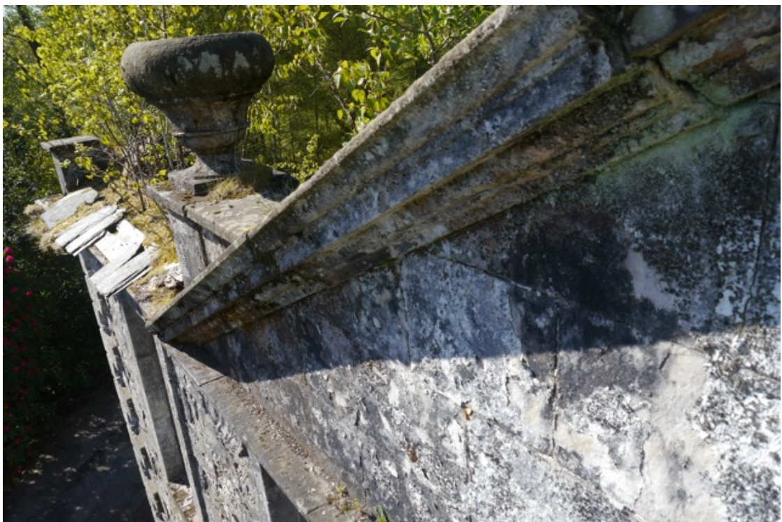
Above and below - pediment stonework is relatively sound.
