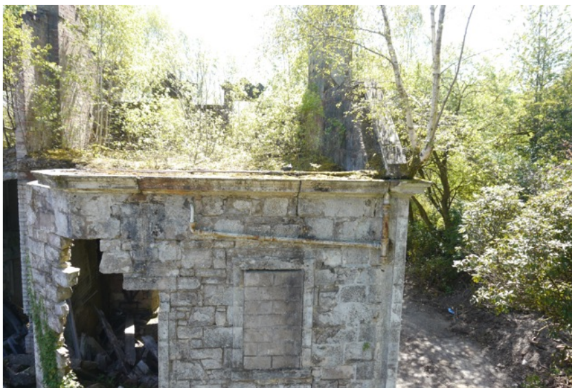
Above - vegetation growing off concrete second floor behind west gable. Left - open mortar joints to west gable.
