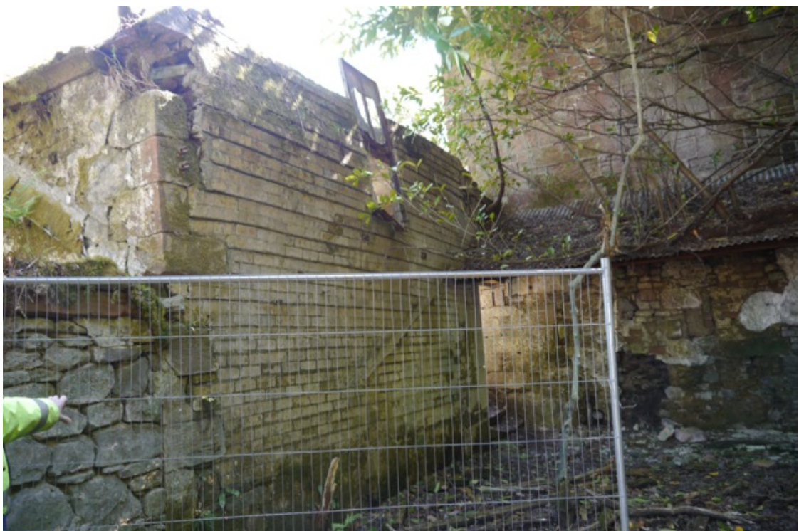
Below - failed end wall of north block.
