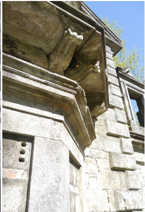
Below - Cracks and open joints to be repointed and plain wall areas lime rendered.
