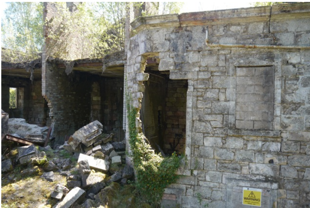
Surviving rear projection - section on left structurally unstable.
