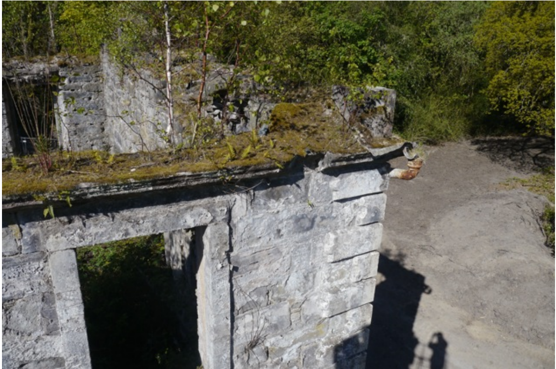
Above and below - vegetation, loose slates and damaged wallhead stonework - the timber boarding is the old sarking - any wallplate would have been set further back.
