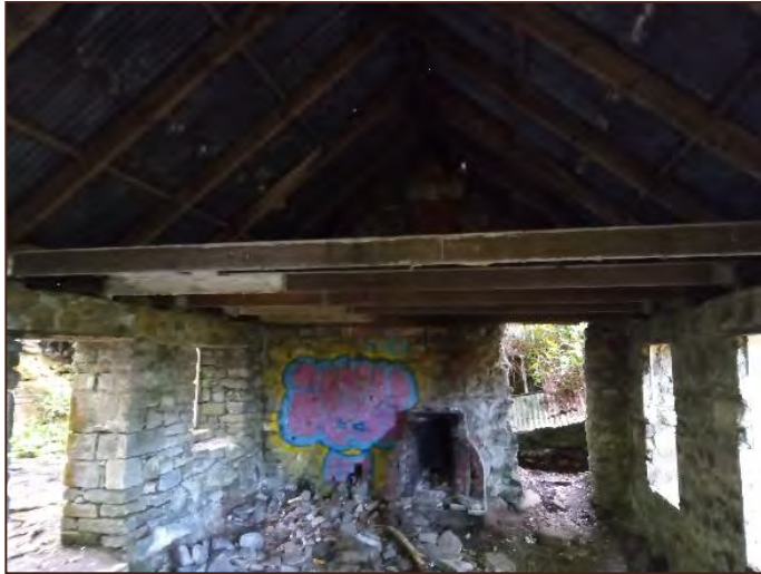
(y) Building C – internal area with single lined roof.
