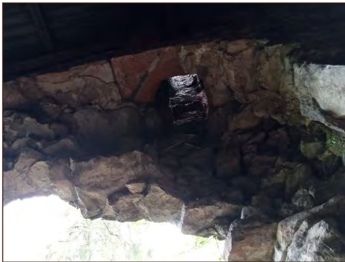
(z) Building C – chimney at the southern end of the building with minimal stone crevices.
