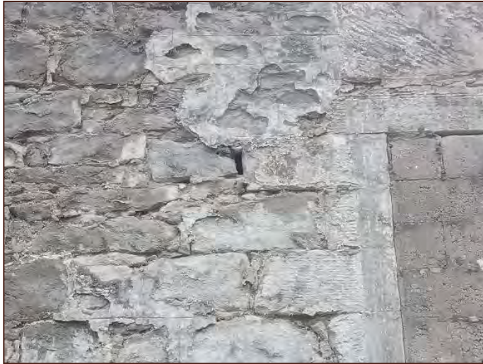
(g) Building A – missing mortar on external wall with deep crevice.
