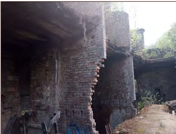
(c) Building A – internal area of the building which had almost entirely collapsed.
