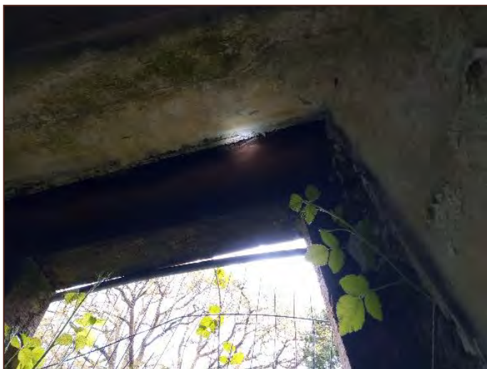
(r) Building B – void within existing window lintels throughout the building.
