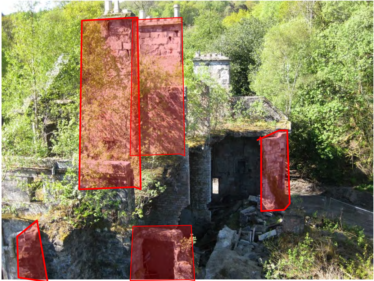
Photograph 6 – View of the walls and slab behind the south elevation (taken from the east) Priority down takings for safety shown in red
