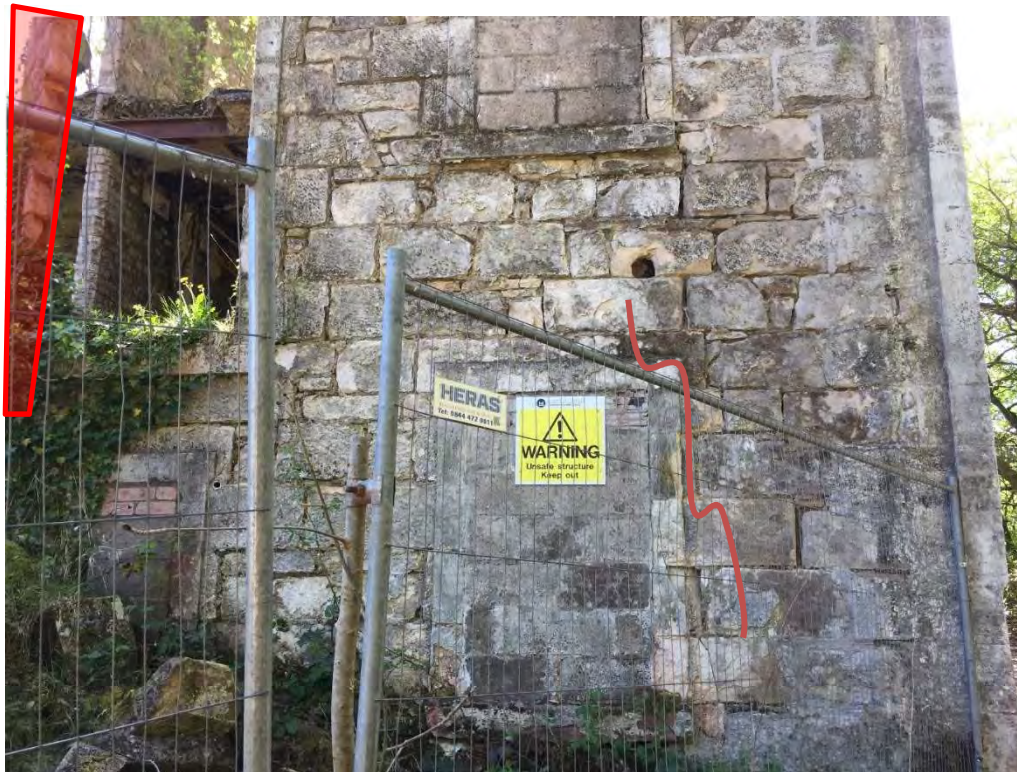
Photograph 9 – North Rear Elevation West low level Priority down takings highlighted red, cracks highlighted in orange.
