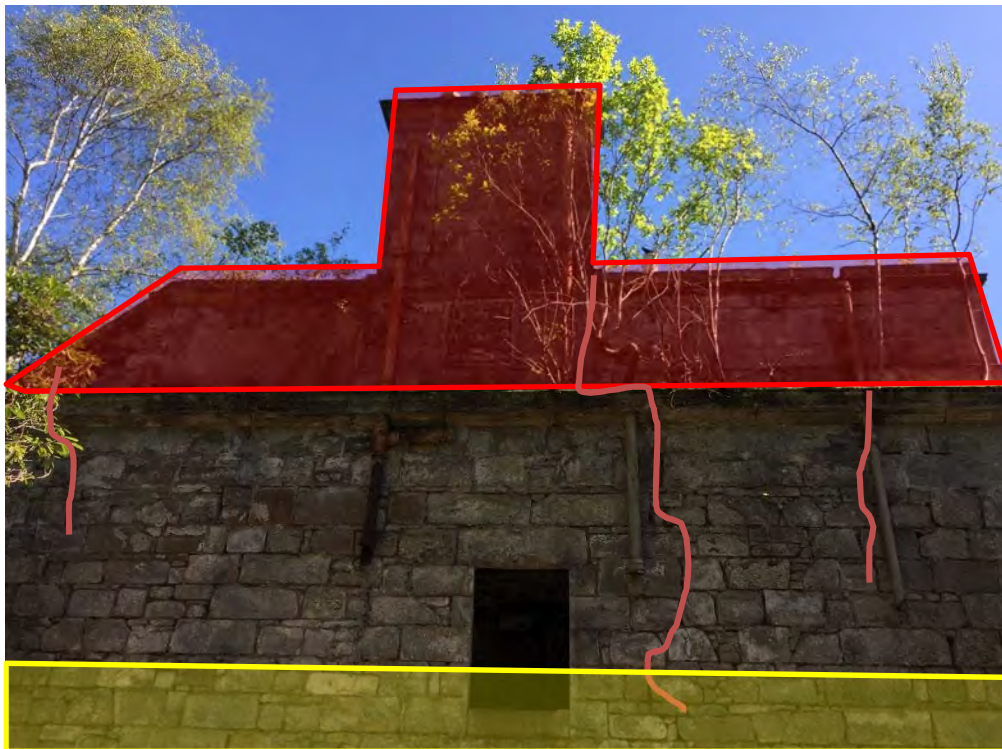
Photograph 7 – West Elevation Demolition highlighted red and badly corroded stone highlighted yellow.
