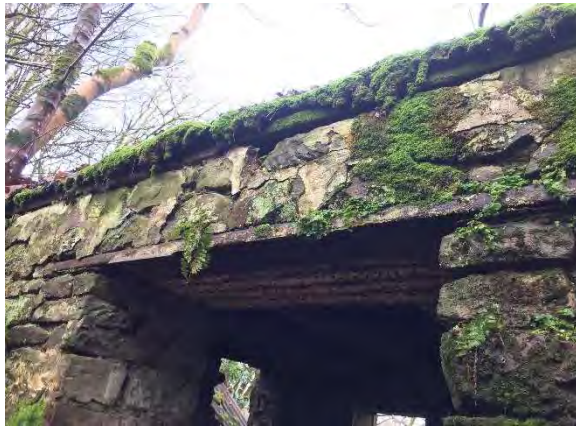
Photograph 31 – West wall lintel, formed with rails
