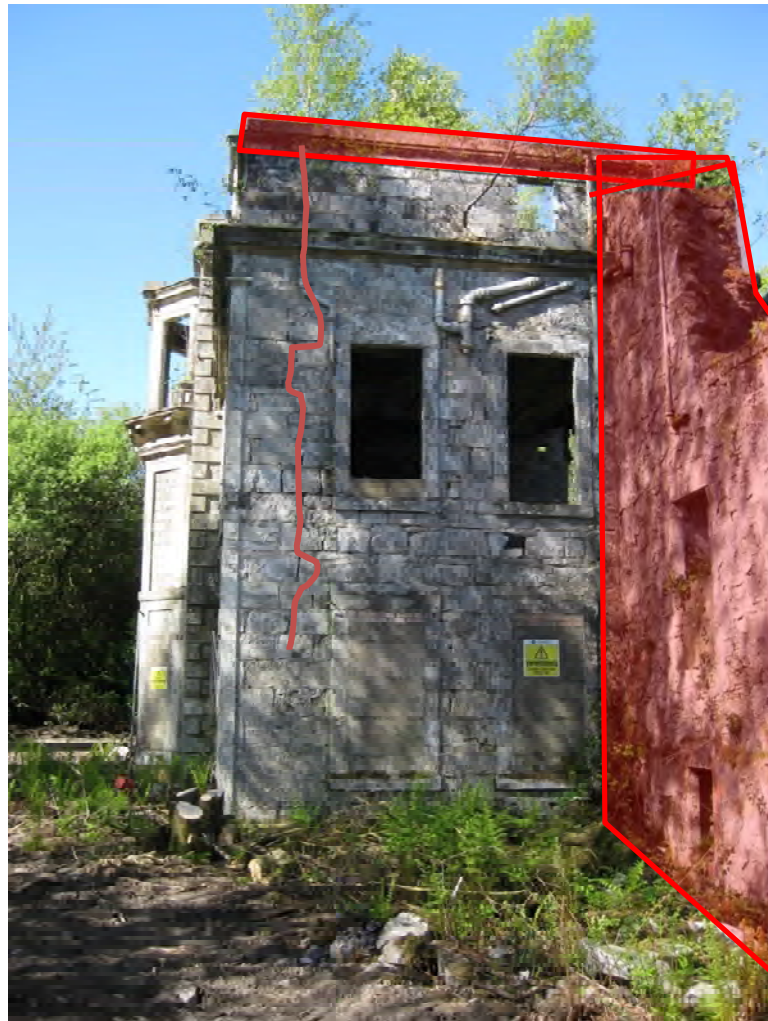
Photograph 4 – Rear East Elevation Down takings shown in red
