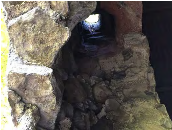
Photograph 29 – South wall, showing unstable flue.
