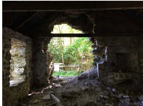
Photograph 32 – South wall, showing collapse.
