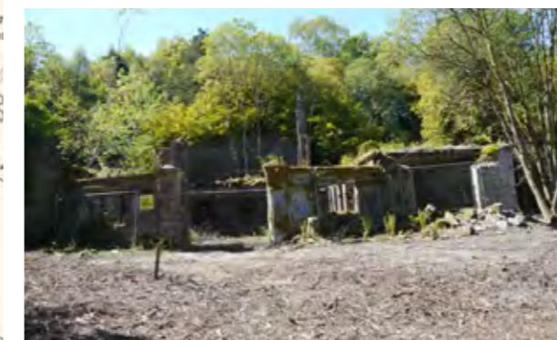
Ancillary buildings - current ruinous condition
