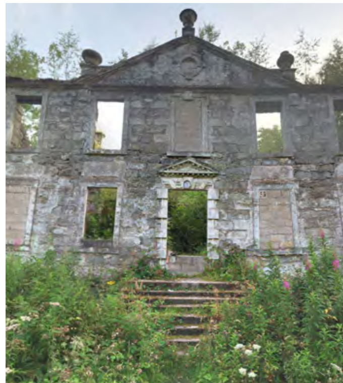
Retain and Restore the listed facade
