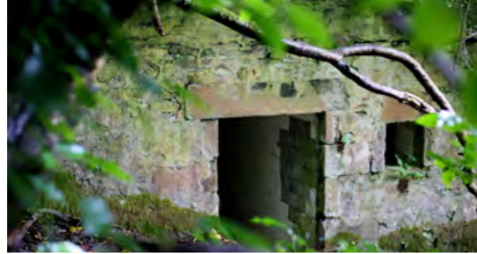
Restoration of derelict buildings
