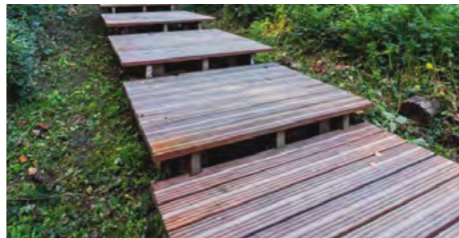
Areas of timber decking for lodges
