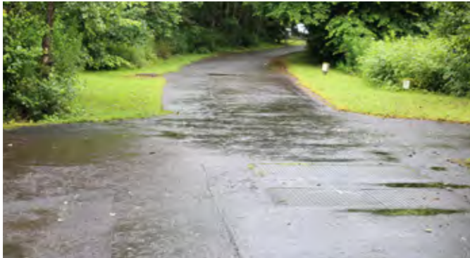
Asphalt along key access routes
