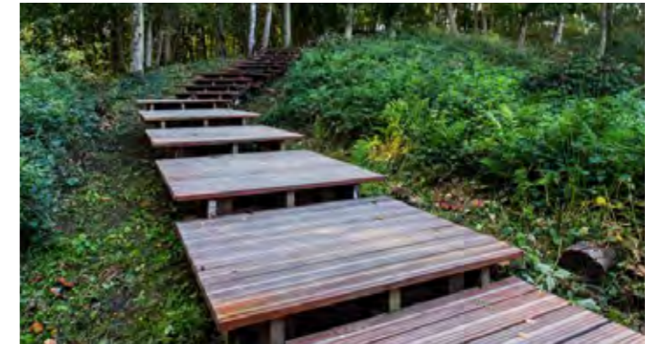
Timber board-walks elevated off ground level
