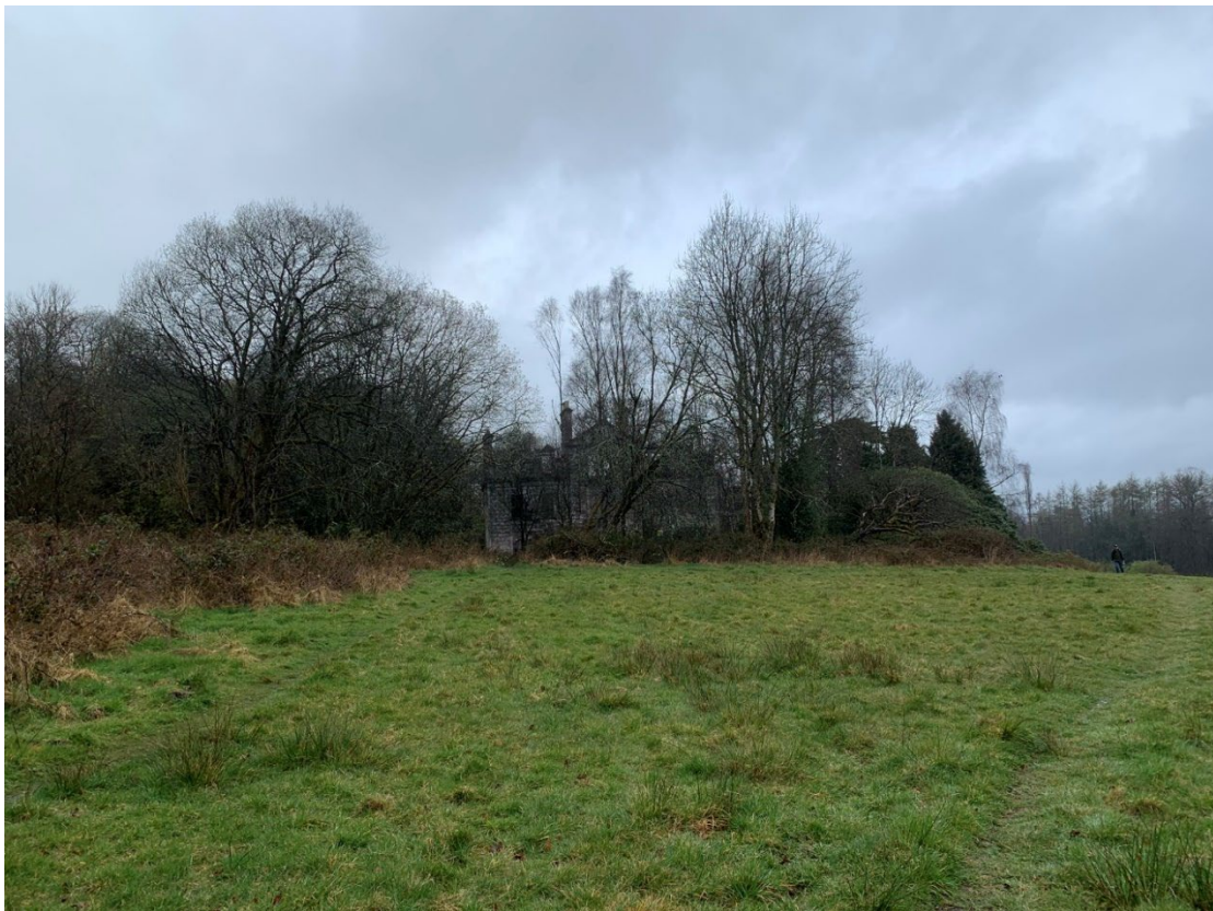
Image 13-2: View NNW of Southern Elevation of Woodbank House from Southern Extent of its Grounds
